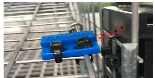
The distance between the magnet and the small hole in the bracket must be less than 10mm.
