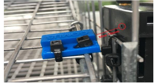
The distance between the magnet and the small hole in the bracket must be less than 10mm.
